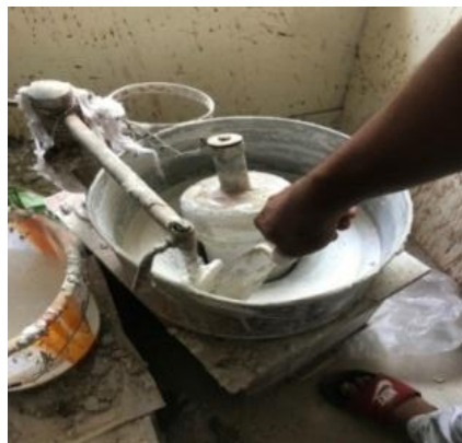
Figure 1 Mixing of lime mortar
