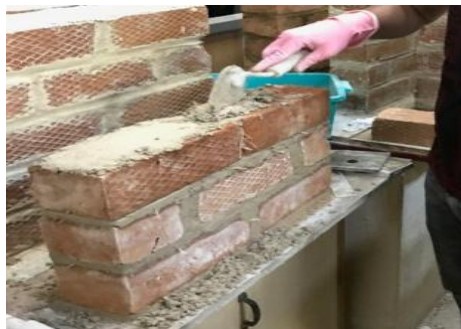
Figure 4 Casting of wall
